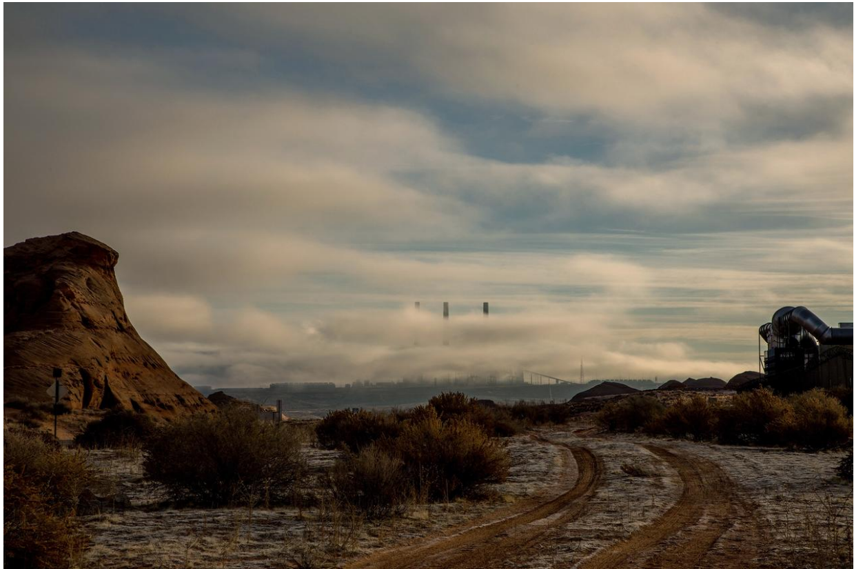
The Navajo Generating Station, January 2020
