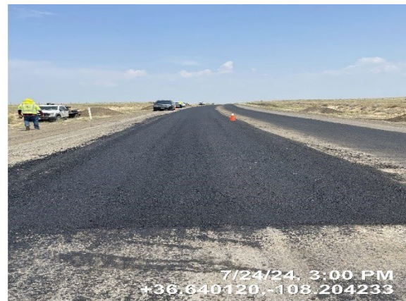
AFTER: New surface on paved road.
